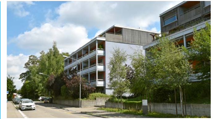
Densification through upwards expansion and renovation of the existing building in order to retain unique structural features (Irchel retirement homes, Zürich, Switzerland).
