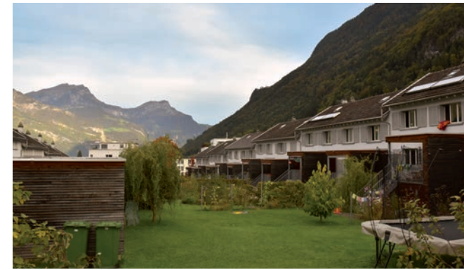
Densification through supplementing with spatial layering, renovation of existing buildings and structuring of free spaces (Turmatt workers' housing development, Altdorf, Switzerland).
