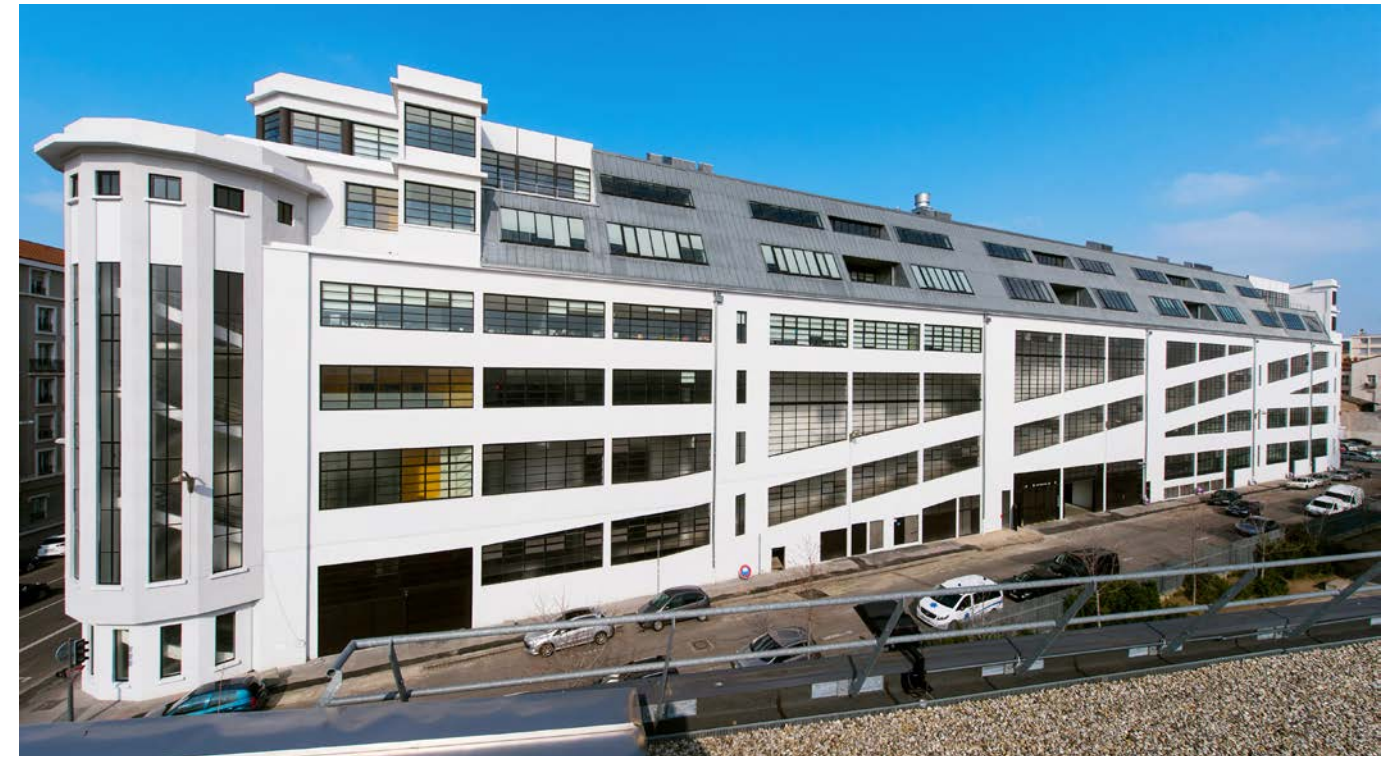
The internal ramps can be clearly seen in the façade on Rue Béchevelin. The small window and fixed glazing sections were reconstructed using Janisol Arte so that they remained true to the original.
