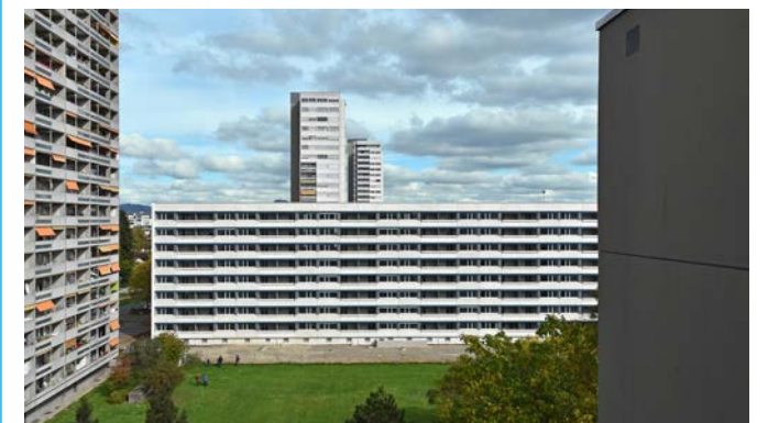
Renovation and supplementation of the existing building with spatial layering to extend the living space in close cooperation with the heritage preservation authorities (Tscharnergut housing development, Bern, Switzerland).
