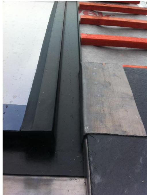
Lead soakers slate profile
